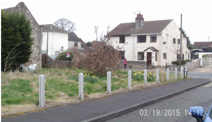
Photos from 2015 application file - Fence posts installed
